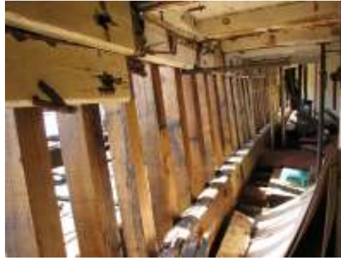
Fig 4 – July 06 – the main frames replaced
