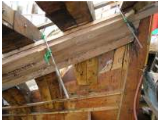
Fig 12 – October 07 – doubled hull planking
