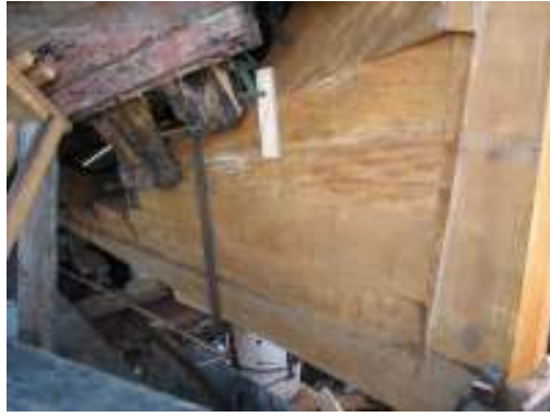
Fig 7 – November 06 – the sternpost and deadwood replaced
