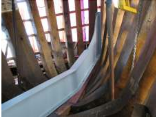
Fig 8 – February 07 – The refurbished central keelson and complex frames at the bow
