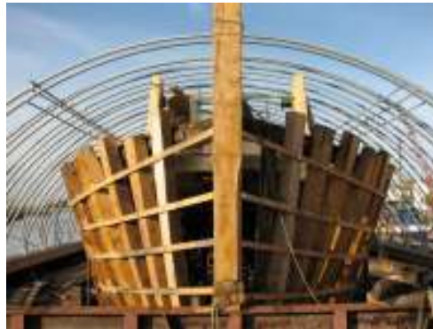
Fig 6 – November 06 – the massive stem replaced and winter shelter in place
