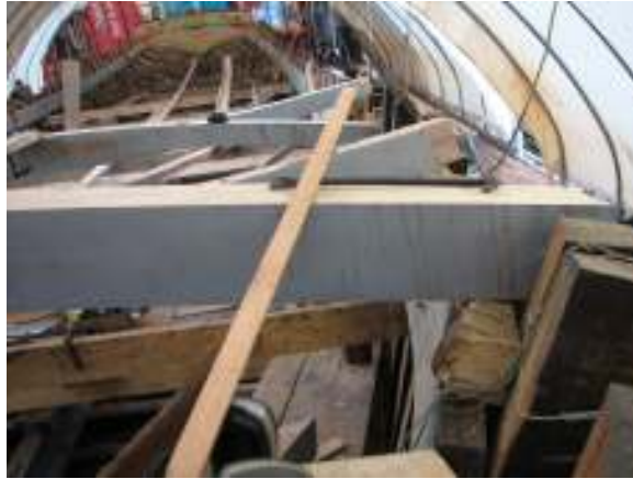
Fig 14 – November 07 - installing the deck beams, looking aft
