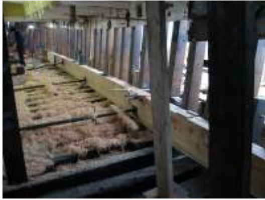
Fig 10 - February 07 – the 50ft chine keelsons being pressed into position
