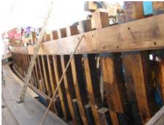
Fig 11 – June 07 – the Whale (side-plank) installed - a key reference for replanking
