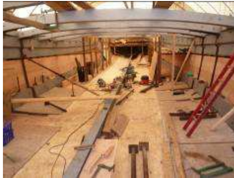
The lining and ceiling installed
