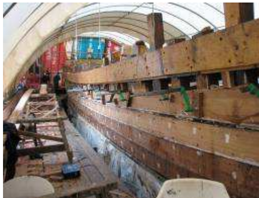
Hull planking nearing completion
