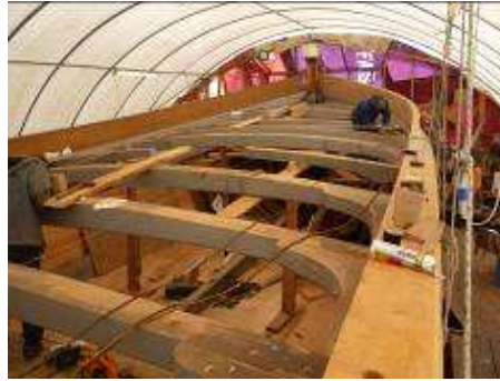
The rail being fitted
