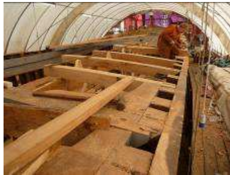
Side deck beams being installed, up to hatch coaming
