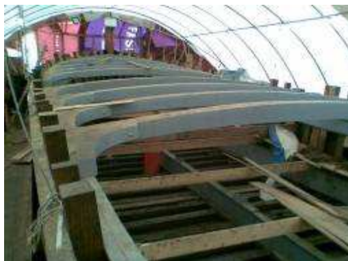
Substantial deck beams installed
